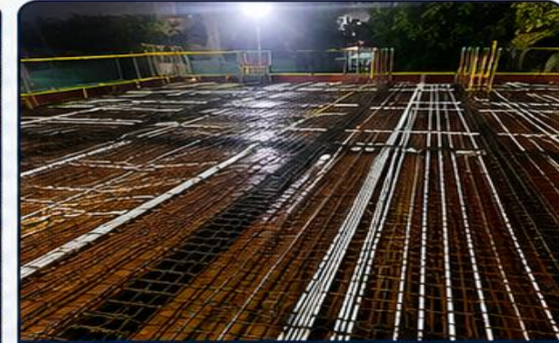
CONDUIT LAYOUT WORK IN PROGRESS
