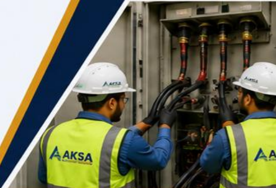
HT CABLE PULLING & TERMINATION
