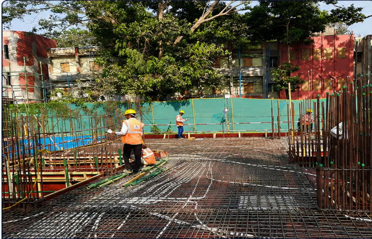
REINFORCEMENT & CONDUIT LAYOUT WORK IN PROGRESS
