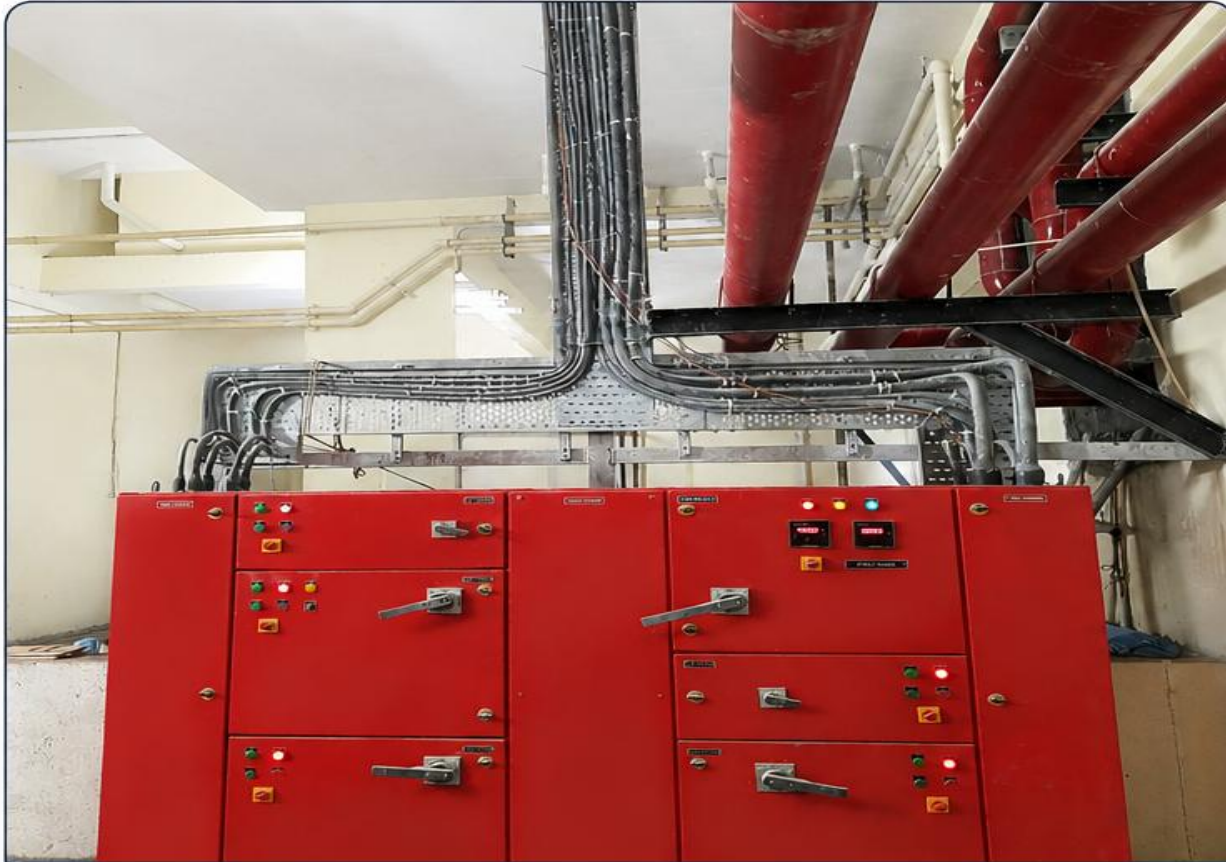
FIRE PANEL & CABLE TERMINATION
