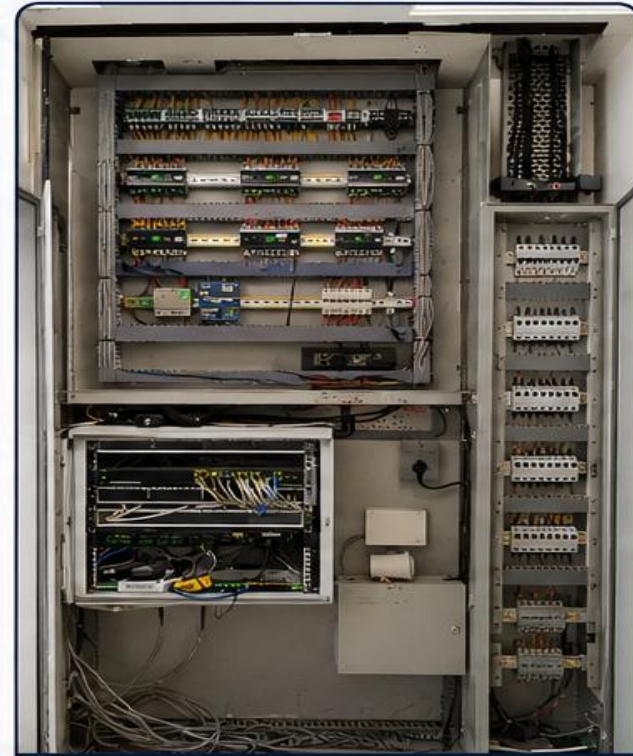
COMMUNICATION & AUTOMATION PANEL
