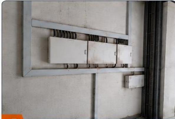
ELECTRICAL DISTRIBUTION PANEL
